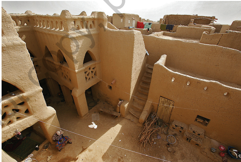
PHOTO 2.7 In Djenné, Mali, people adapt to the hot mostly dry climate by building houses in adobe. The picture shows the inner courtyard of a Djenné house. Thick walls keep rooms relatively cool in the hot season and warm when it's cold. Flat roofs create more living space and can be used for sleeping during hot weather.
