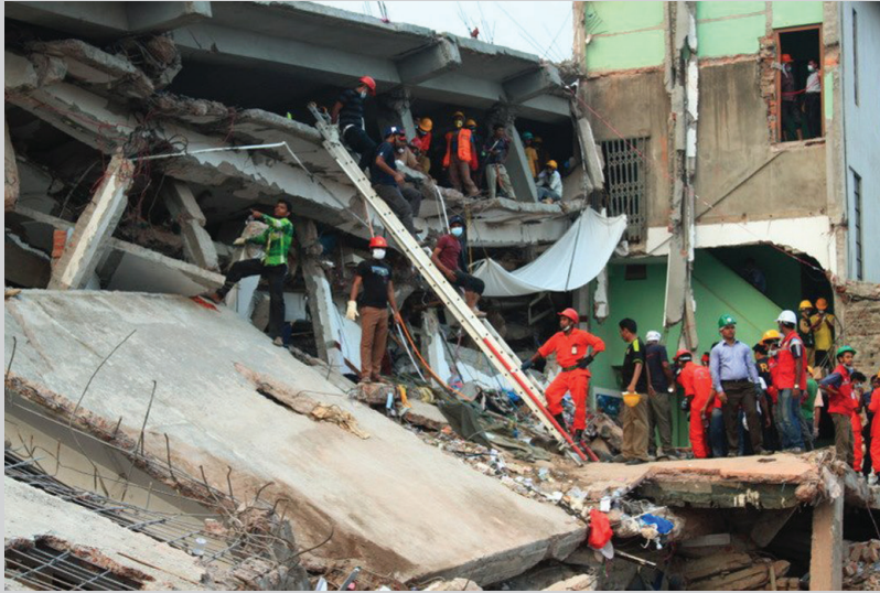
Dhaka garment factory collapse in Bangladesh
