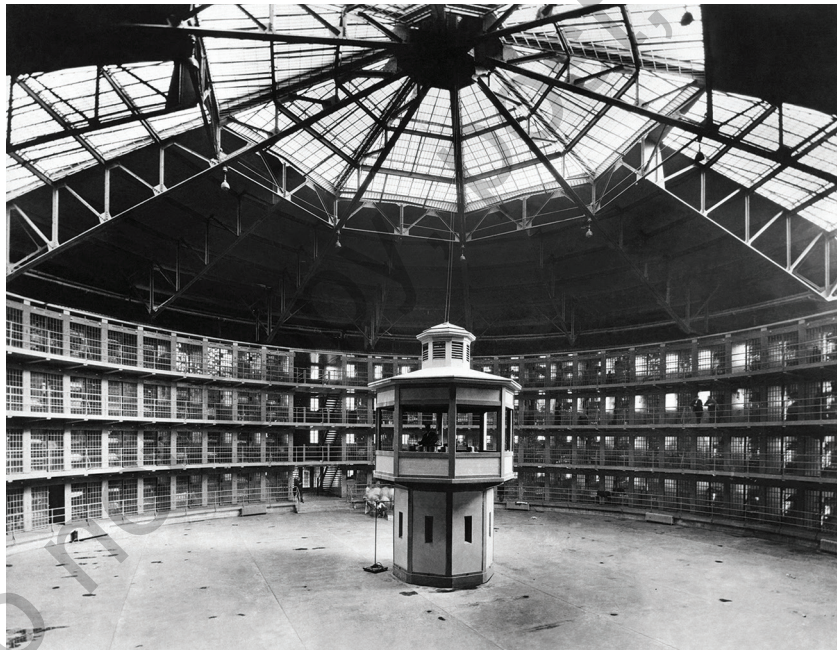
PHOTO 2.4 Stateville Prison in Illinois was built as a panopticon, with rounded architecture and a central tower for officers. Panopticons were devised to enhance the supervision of inmates but may have been more effective at enhancing the observation of officers by inmates.
